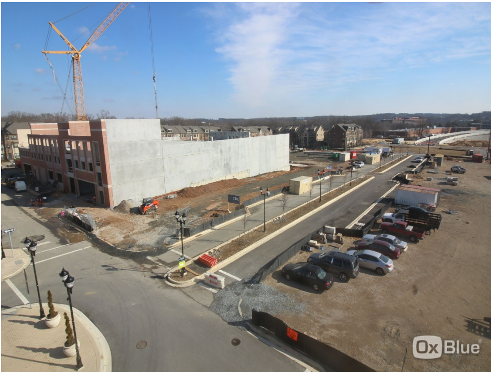
Picture Below: Building 5 Parking Garage Progress – Precast Walls Installation
