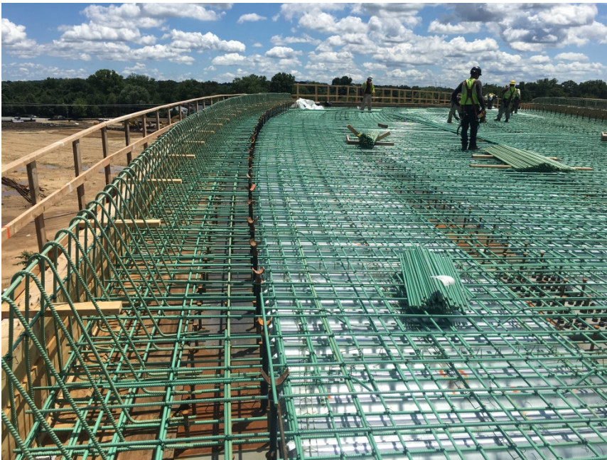
Picture: Bridge Deck – Looking East: July 2017
