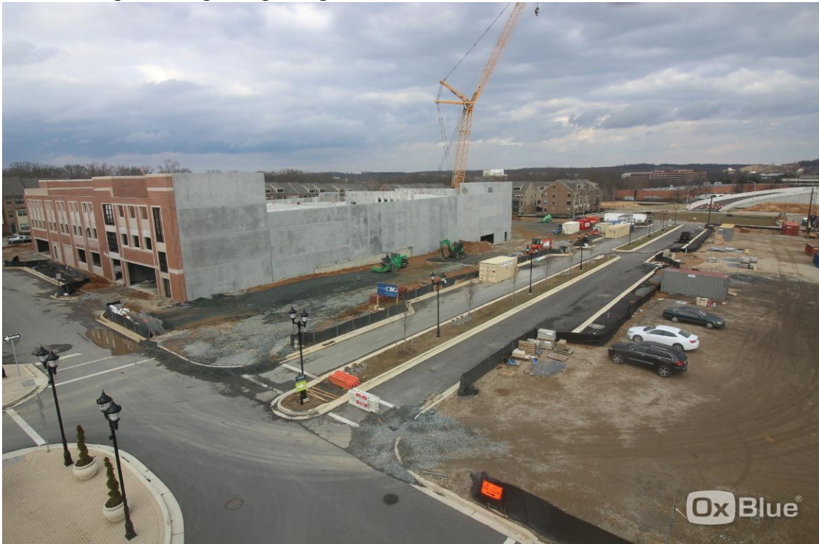
Picture Below: Building 5 Parking Garage Progress
