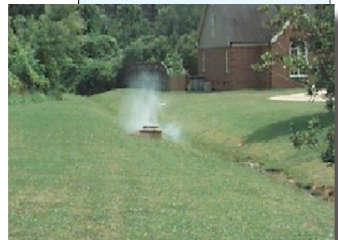
Smoke exiting the sewer system
